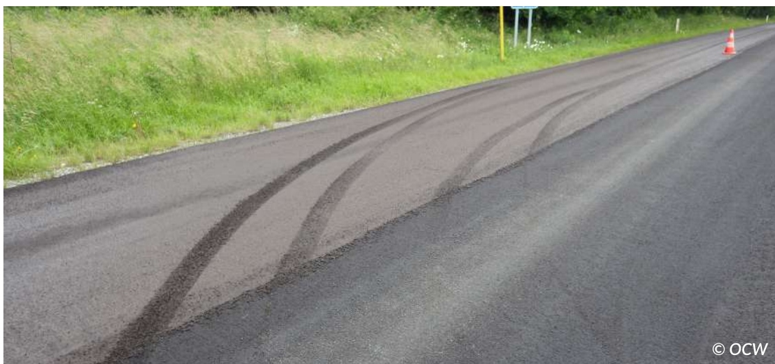
Figuur 6.6 – Bandenspoor in verse slem
