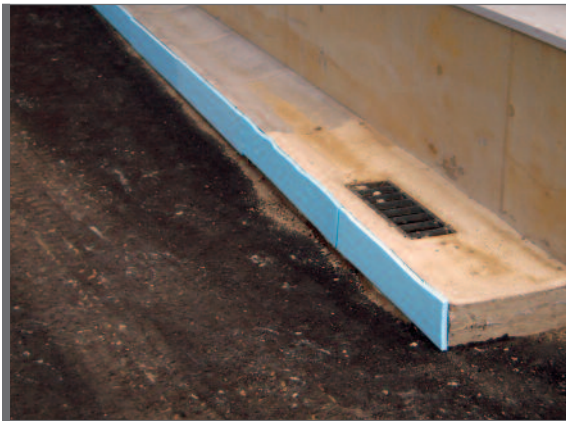
Figure 3.2 Joint de dilatation/isolation
